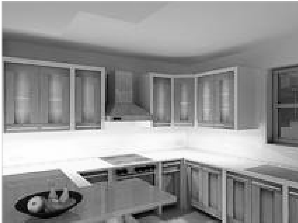
Under-cabinet lighting using 14W and 28W T5 linear fluorescent lamps Source: www.gelighting.com
