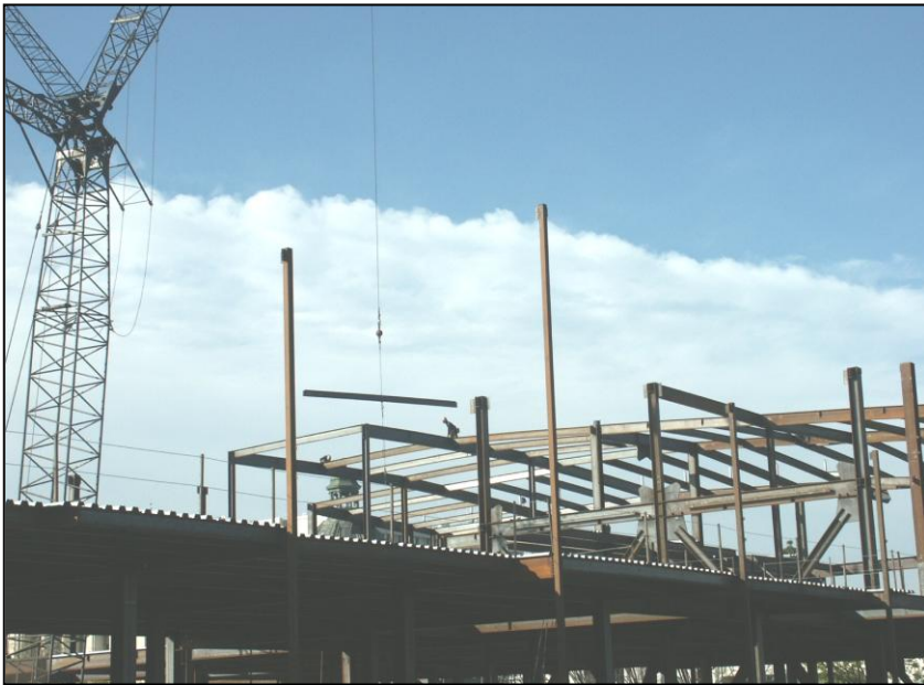
Construction of Downtown “On Broadway” Retail/Cinema Project
