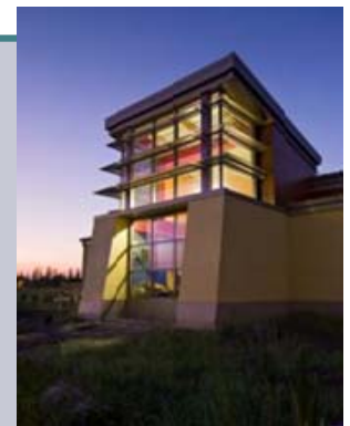
Redwood Shores Branch Library
