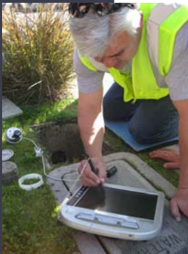
Water crew installing a new water meter
