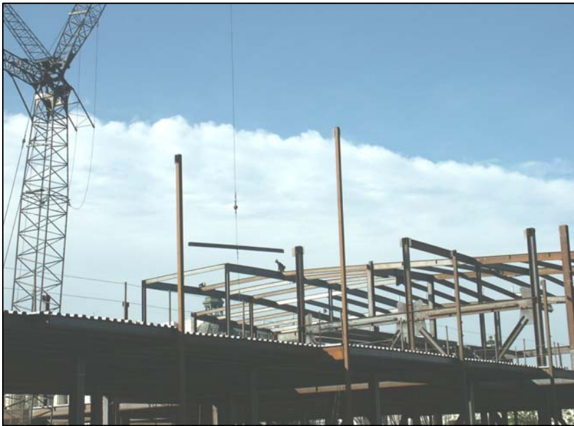
Construction of Downtown “On Broadway” Retail/Cinema Project
