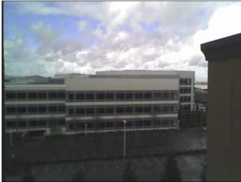
View towards project from adjacent apartment building. Closest, northeast wing of 420 Broadway is in center, southwest wing of 420 Broadway is on the left, and 430 Broadway is further away on the right. (Photo provided by applicant.)
