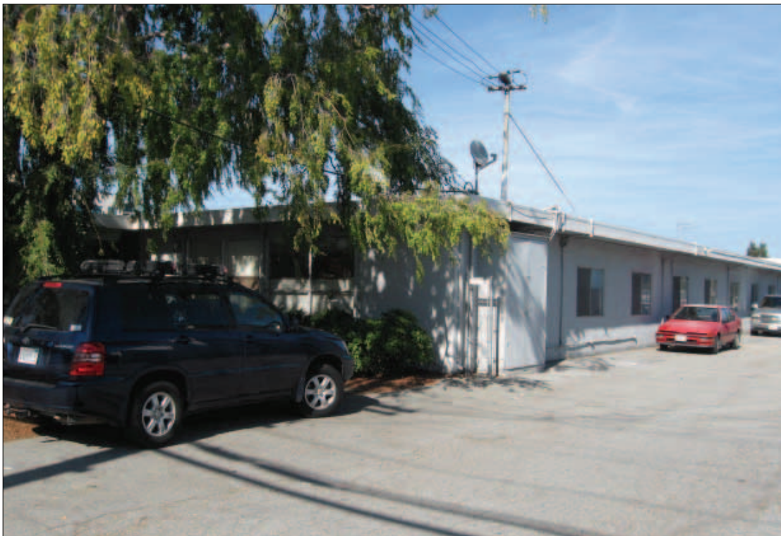
Photo 2 - View of the on-site office building, looking northeast from the southwestern boundary of the project site.
