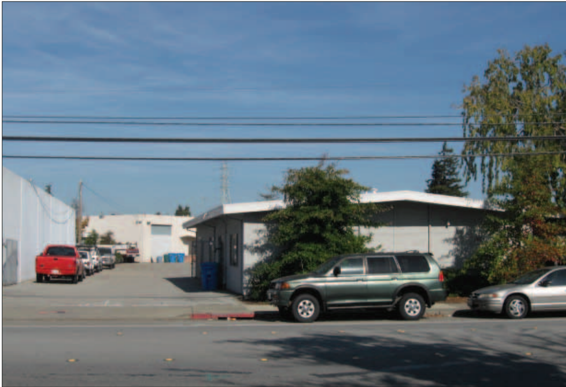
Photo 3 - View of the project site, looking east from the western side of Industrial Way.
