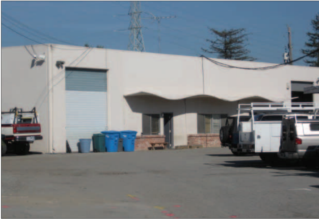
Photo 1 - View of the on-site warehouse building, looking east from the northern boundary of the project site.
