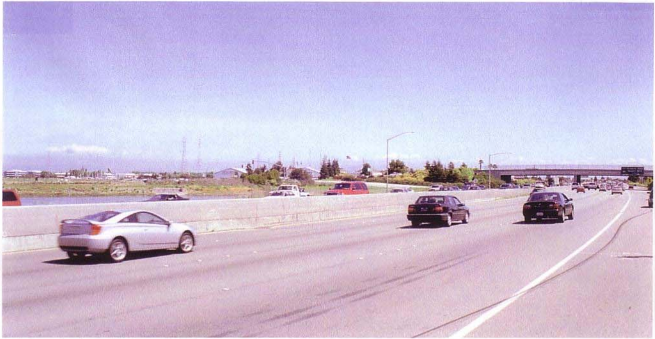
Existing view from Highway 101 southbound near Whipple Avenue
