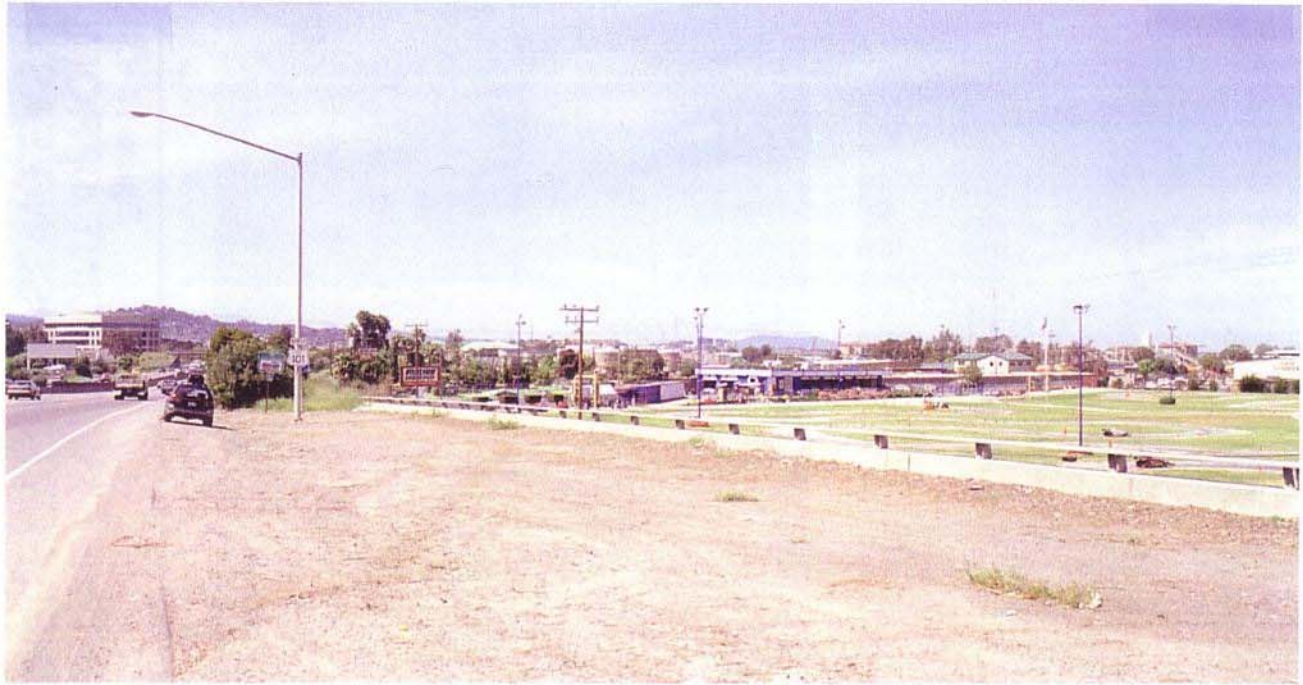
Existing view from Highway 101 northbound near Seaport Boulevard onramp
