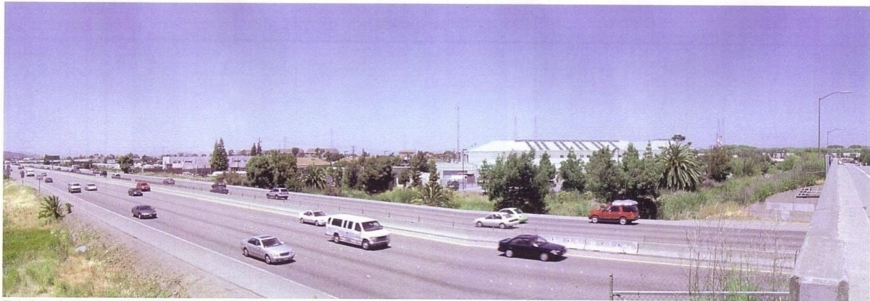
Existing view from Maple Street overcrossing
