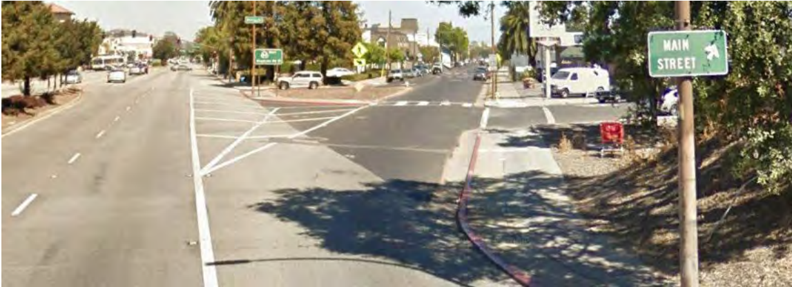
Crosswalk at El Camino Real/Main Street-Spruce Street. Intersection geometry that lends itself to higher vehicle speeds may result in crosswalks that are inconsistent with meeting safety objectives for pedestrian crossings.
