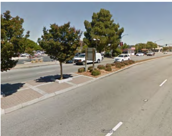
Medians vary in width and utility, providing tree coverage and landscaping where wider and channelization where narrower.
