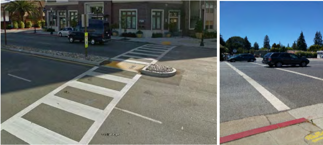
A high-visibility ladder-style crosswalk across the south leg of El Camino Real/Northumberland Avenue provides a pedestrian refuge via a break in the raised median island (left). A standard uncontrolled crosswalk across El Camino Real (ECR) located on the south leg of ECR/Edgewood Road, on the other hand, forces pedestrians to cross approximately 70 feet without refuge from vehicle traffic (right).
