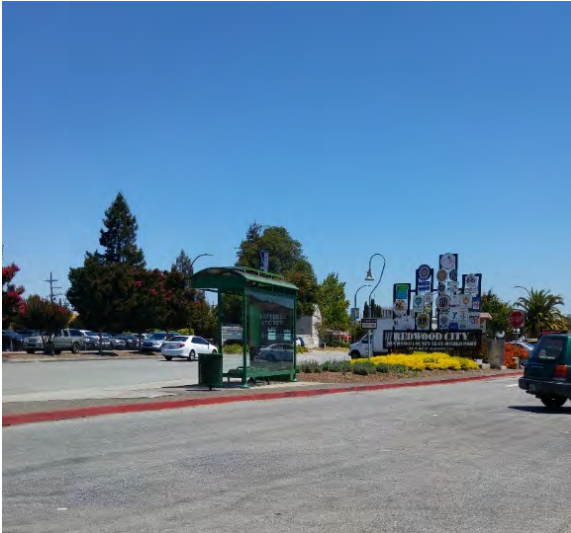
Southbound bus stop at El Camino Real/Claremont Avenue, view looking southeasterly. Pedestrians must cross the frontage road to access the bus stop raised island, with curb ramp access via a concrete shoulder that is not delineated or otherwise separated and is at grade with El Camino Real to the right of the travel way. Pedestrian facilities are discontinuous.
