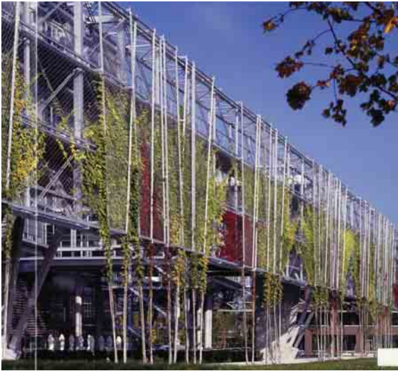
Facades facing open space areas may include exterior stairways and an integrated green wall system.
