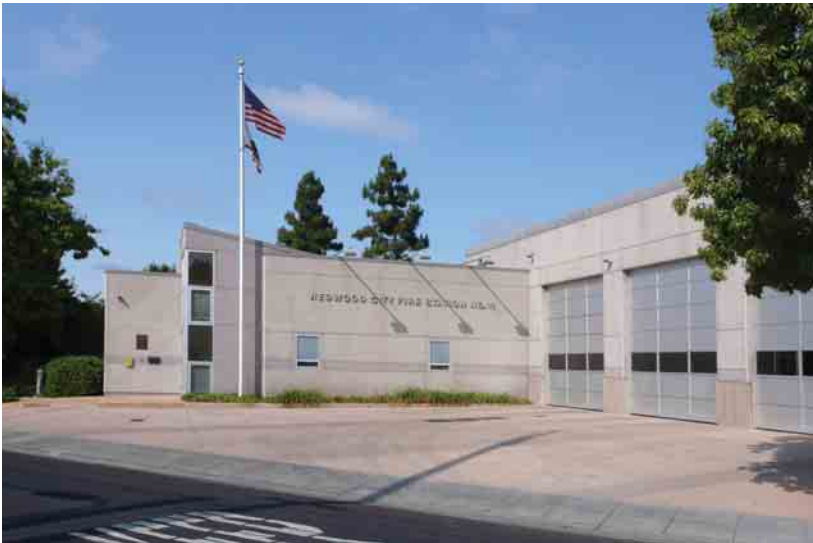
View of Redwood City Fire Station 11.
