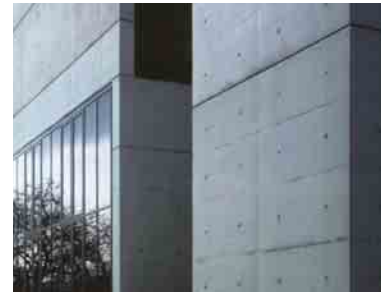
Cast in place concrete
