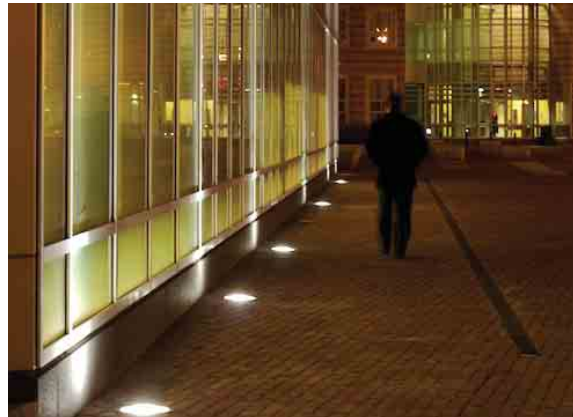
Consistent lighting fixtures should illuminate the path without becoming a strong element in the landscape. At-grade lighting is recommended where lighting levels can be minimal.
