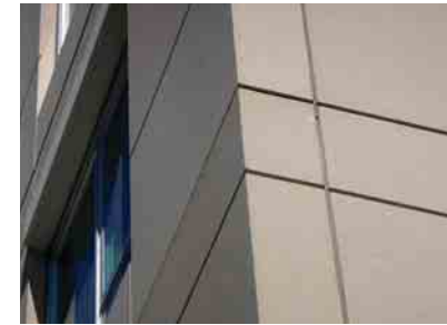
Pre-cast concrete / GFRC pannels
