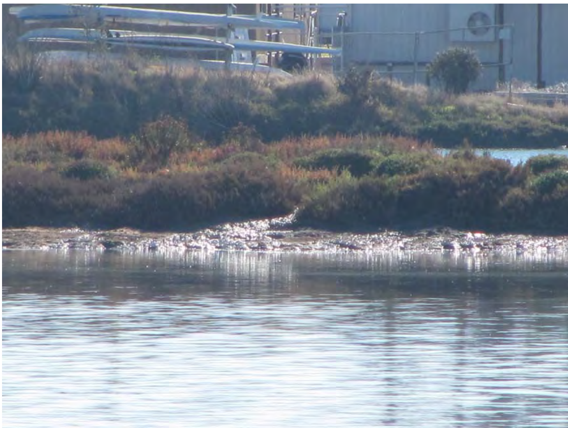
Ferrari property diked wetland showing mudflat and pickleweed on inboard side of levee. Steinberger Slough is in the background just beyond the levee. November 9, 2014
